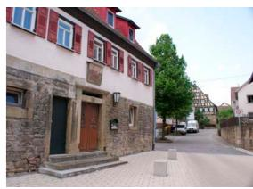
SANDSTEIN ALS SOCKELZONE ODER MAUER
