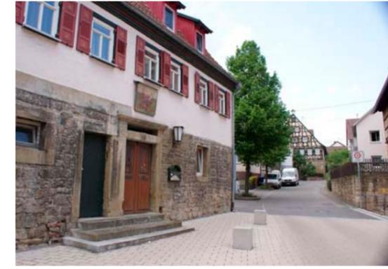
SANDSTEIN ALS SOCKELZONE ODER MAUER
